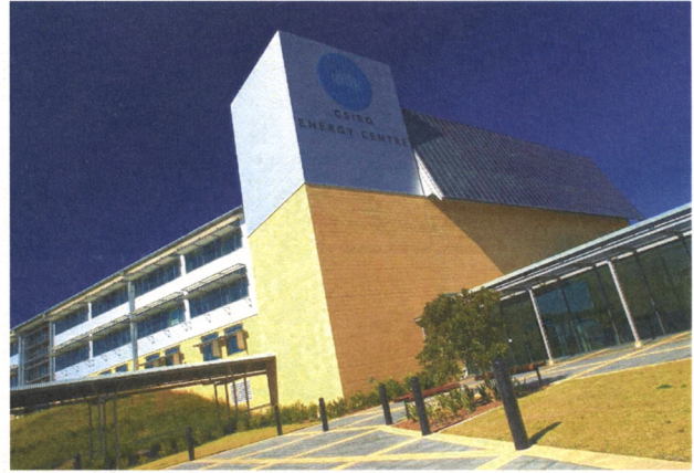
Figure 3: CSIRO Energy Centre, Newcastle.
